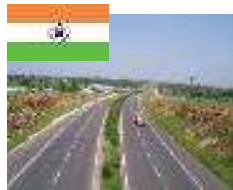
East-West Corridor Uttar Pradesh, India Completed: 2008 Value: US$67 mil
