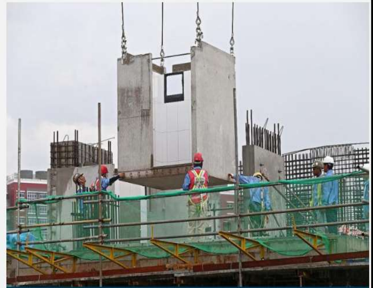
Prefabricated bathroom units are assembled with finishes in a factory before it is transported to a construction site for installation.
