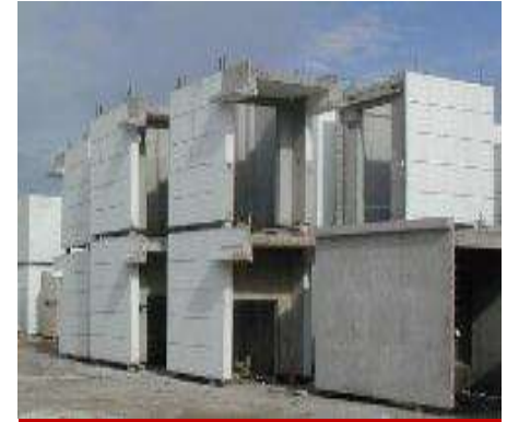
Lift Core Wall
