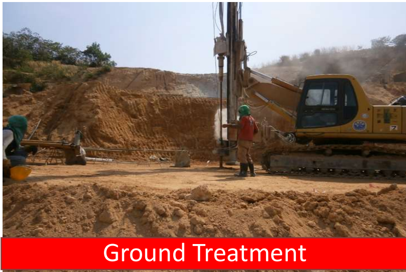
Pile Foundation Works
