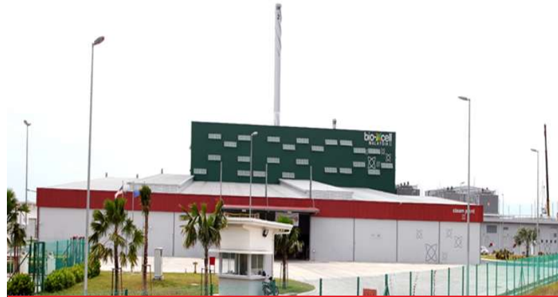
Central Utilities Facilities
